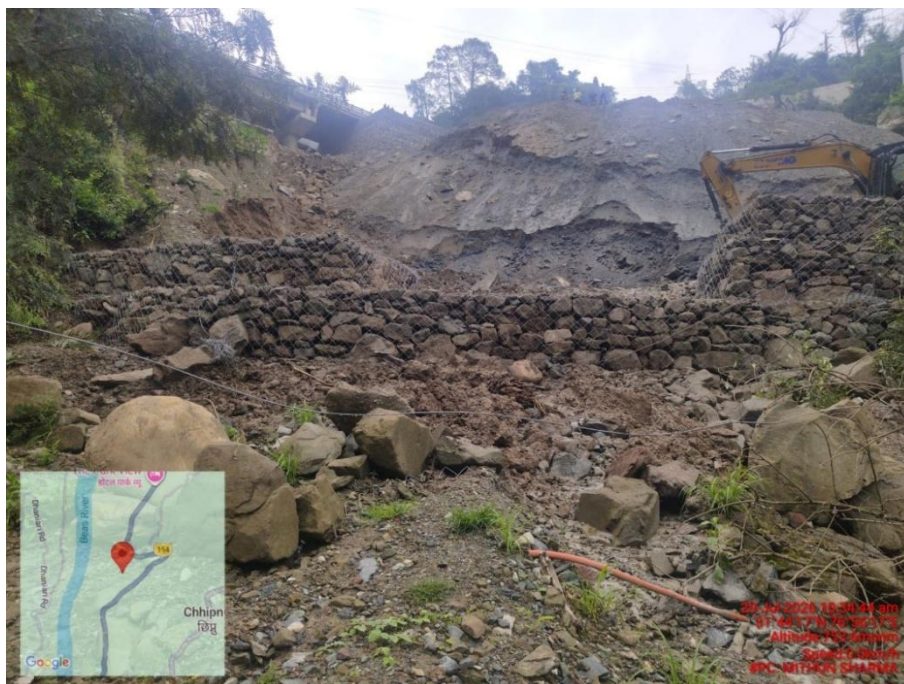
Protection provided Near P-1 Portal at Bijani
