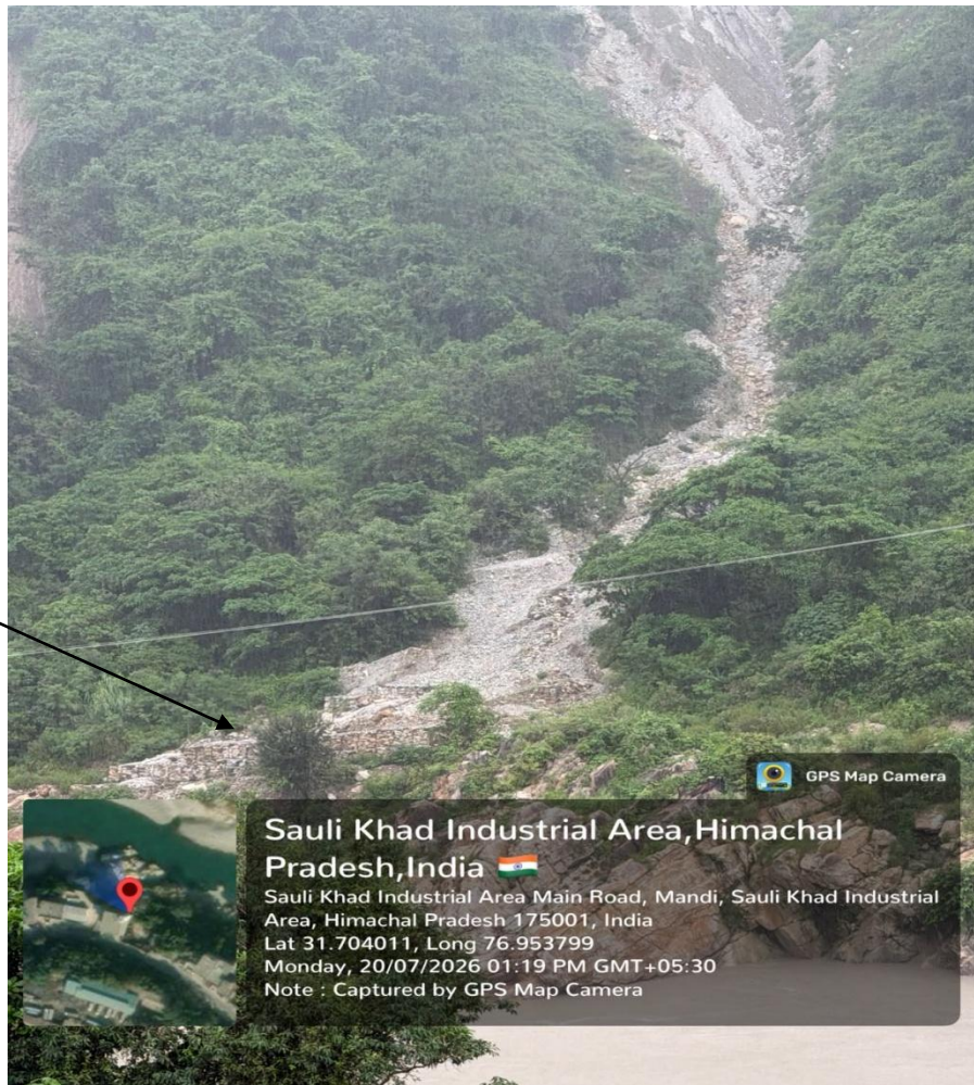
Protection provided at Non designated Site No. 02
