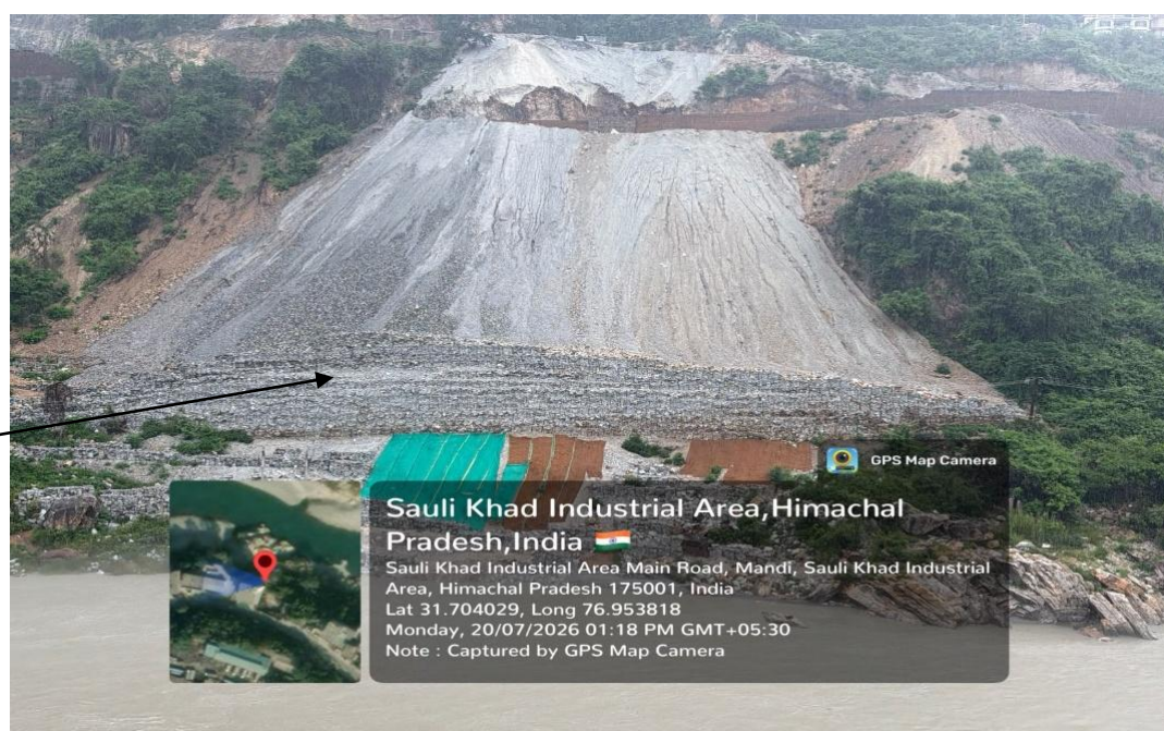
Protection measures provided at Site no. 01.
